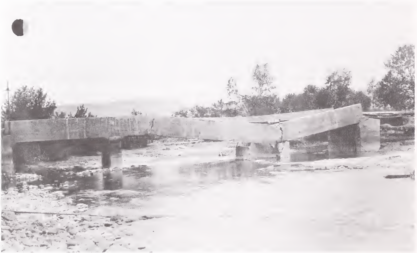
In June, 1917, the reinforced concrete slab bridge over the Boulder River south of Boulder failed during spring run-off. The river undercut one of the piers causing the bridge to settle into the water (Montana Historical Society).
